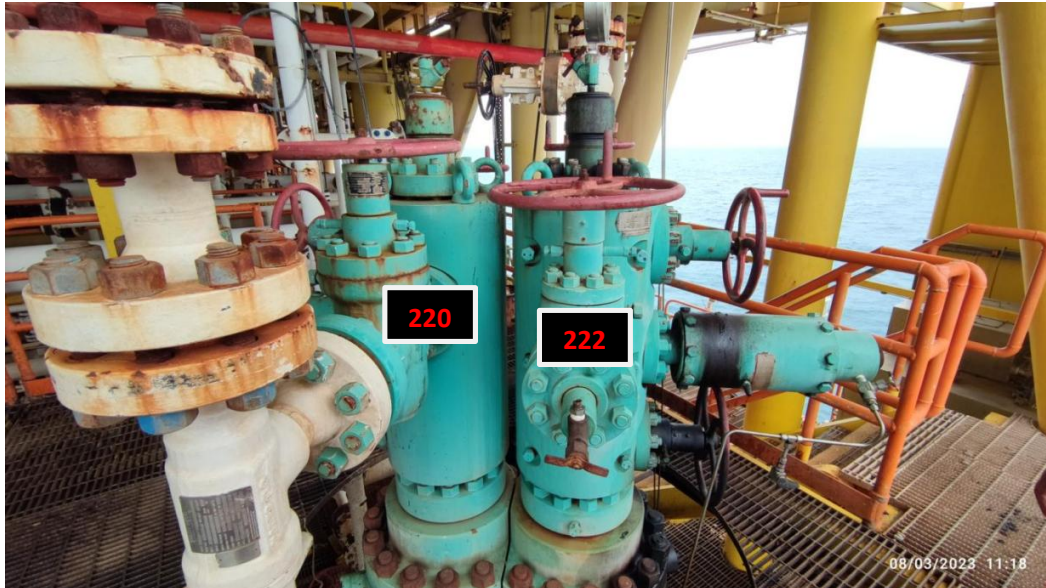
Fig: X-max tree well By-220 & By-222
