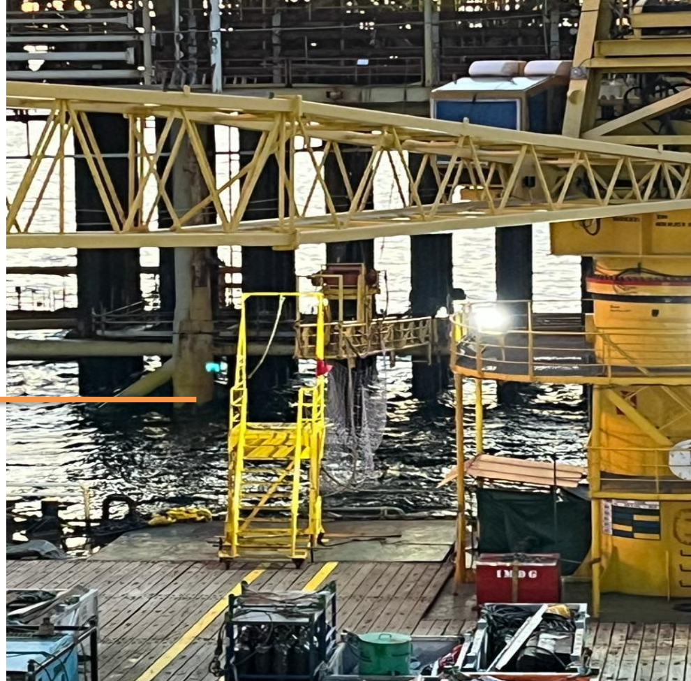
Figure 5: Location of Personnel Transfer for interrig/mob from work barge
