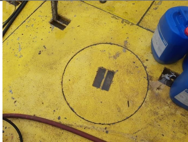
Fig: Plate Cover C08. Diameter: 2.5 ft
