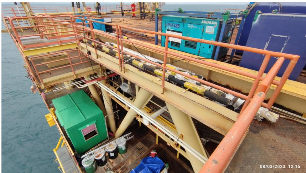
Fig: Overview of loading bay.
