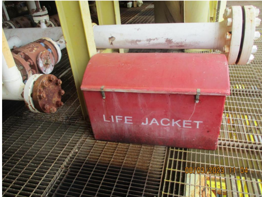
Fig: Life jacket box at cellar deck.
