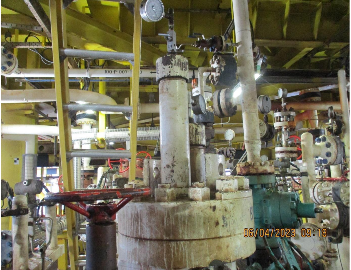
Fig: X-mas tree well BN-49 L/S.
